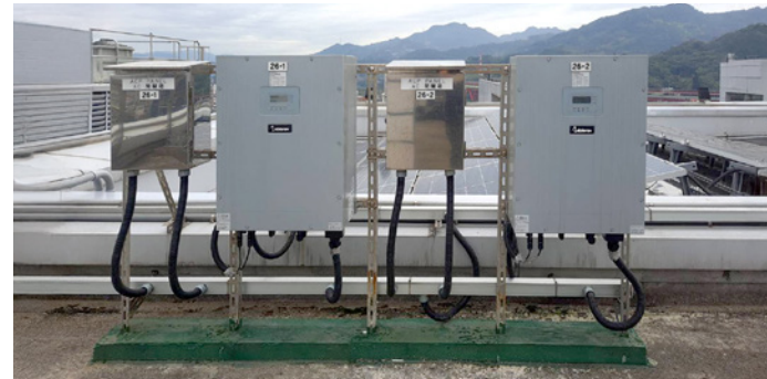
◆ Solar power inverters on the rooftop of our Baogao Science Park building.
